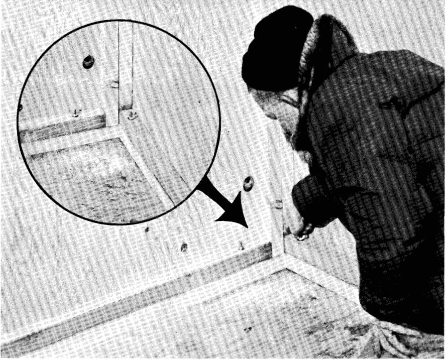
Figure 3.—Wing nuts are used for rapid assembly of the instrument shelter.
