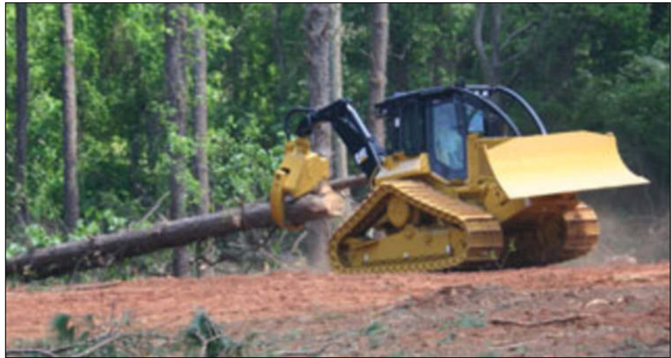
Figure 4. —Medium-size, track-mounted crawler dozer with grapple in back and blade in front skidding a turn of logs (photo courtesy of Caterpillar).
